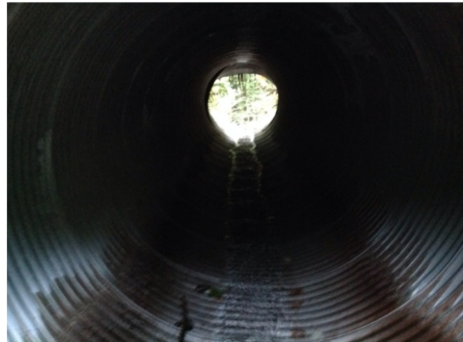
looking thru left culvert
