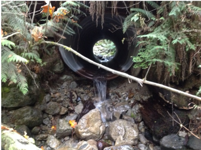
outlet of left culvert
